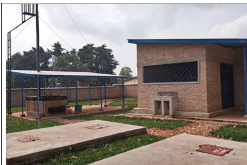
Muyinga District Hospital Incinerator, Burundi
