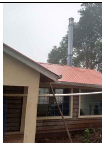
Marsabit Hospital incinerator, Kenya
